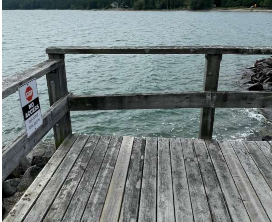
Photo 11: Loose Guard at Viewing Platform
