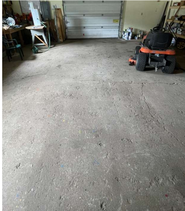
Photo 5: Extensively Cracked and Spalled Concrete Floor Slab
