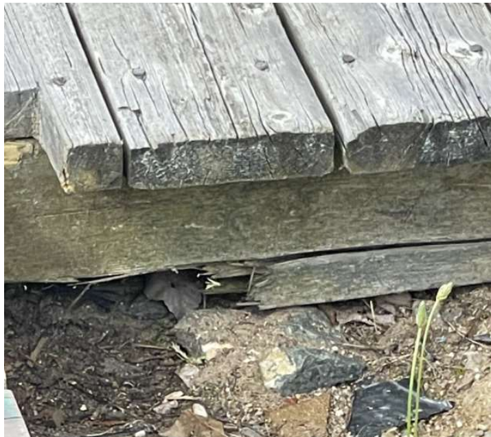
Photo 5: Deteriorated Wood Construction on Boardwalk
