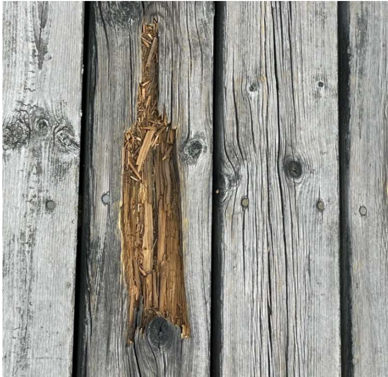
Photo 9: Decayed Wood on Boardwalk
