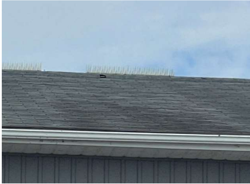
Photo 5: Heavy Organic Staining on Asphalt Shingles
