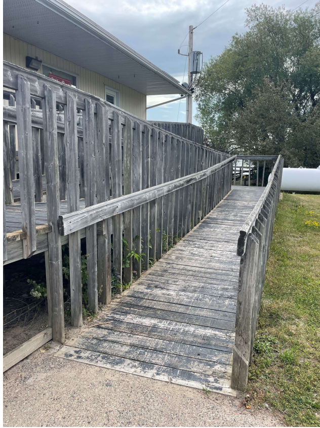
Photo 3: Weathered and Decayed Wood Ramp at Entrance to Canada Post
