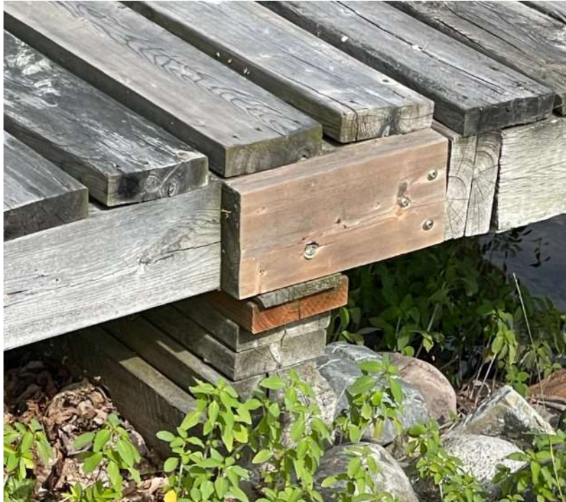
Photo 6: Wood Shim Support on Underside of Dock Structure
