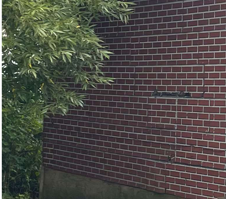
Photo 5: Asphalt Brick Siding Panels
